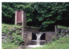
(a) Concrete dam and weir
